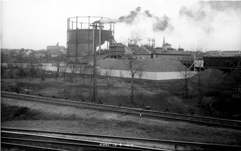
*Northwestern Gas Light and Coke Company, Blue Island, IL 1912. The gas holder is the tall cylinder on the left. The gas holder had a floating cover that rose and fell as the volume of gas increased or decreased. Coal storage is on the right behind the fence. This picture was taken by MWRD as part of the route survey for the Cal Sag Channel. MWRD photo.*
