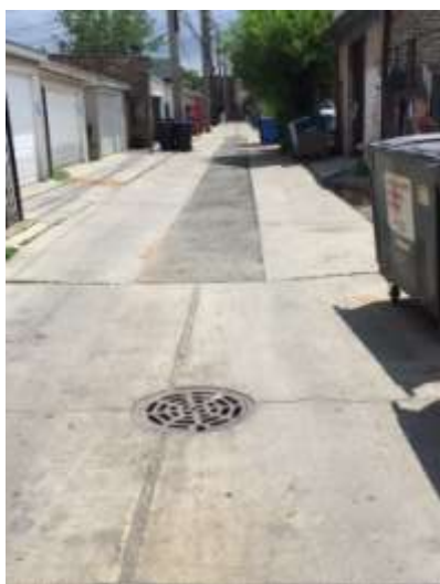
Hybrid Alley – Regular concrete wheel paths sloped to permeable concrete with overflow catch basin
