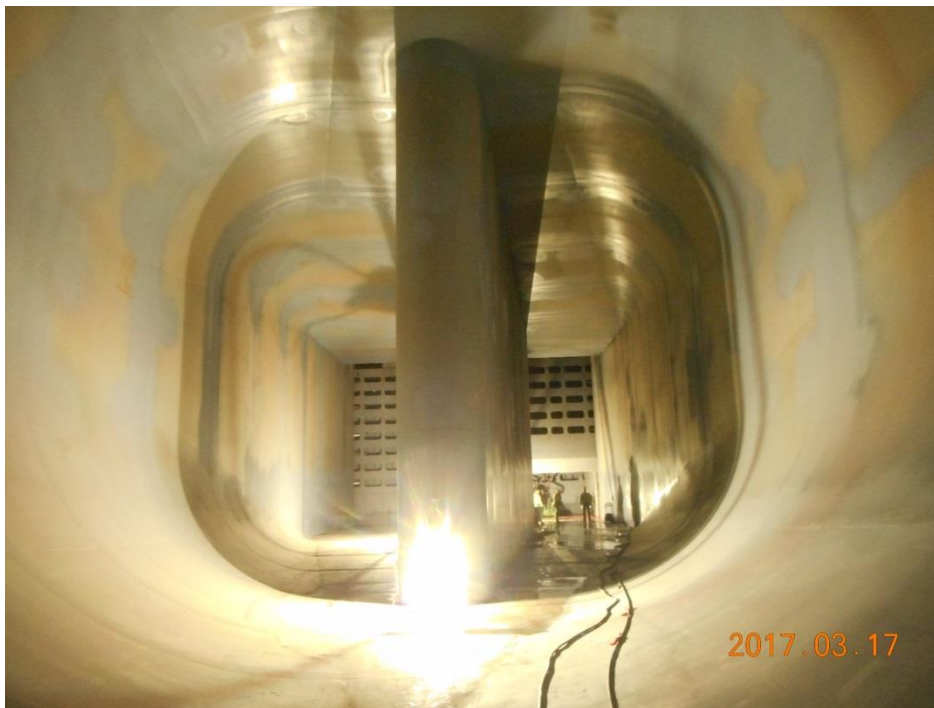
Bifurcated Steel-Lined Section of the Main Tunnel and Gates
