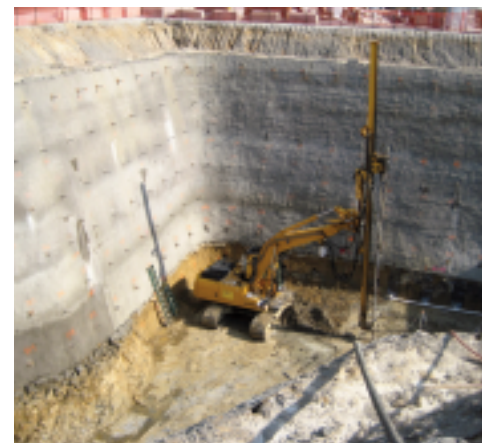
Figure 8. Photograph of excavation through 6 rows of nails.
