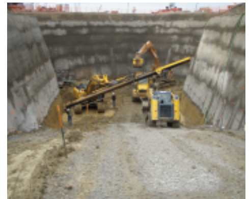
Figure 7. Photograph of the soils nails being installed on the ramp.
