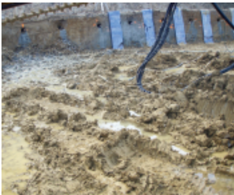
Figure 5. Photograph illustrating wet conditions after the first lift excavated.
