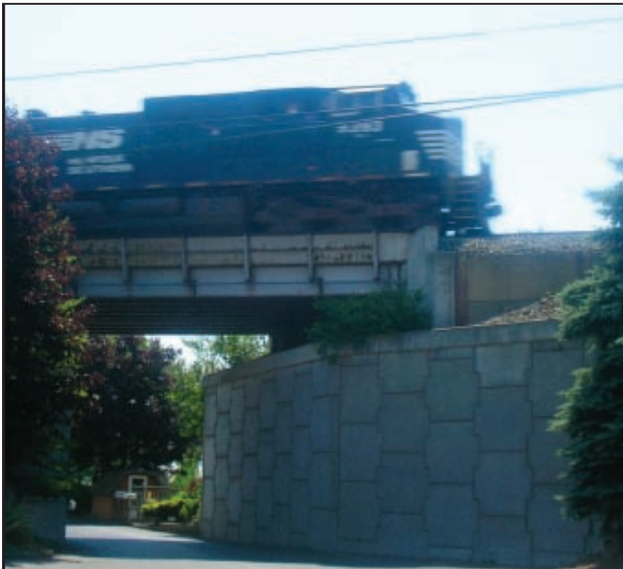
Conrail UG Bridge 183 for Conrail, Cleveland, Ohio. Constructed in 1984
