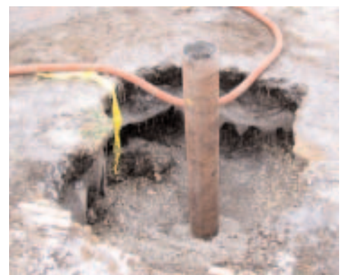
Figure 4. Installed Micropile within Cofferdam Cell
