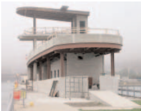
Figure 2. Lock House during Construction
